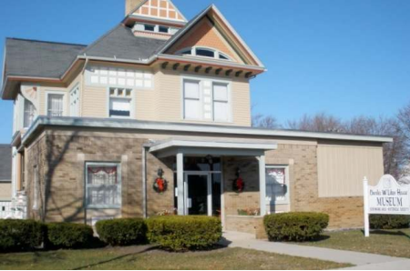
Charles W. Liken House 325 N. Center Street , Sebewaing .
